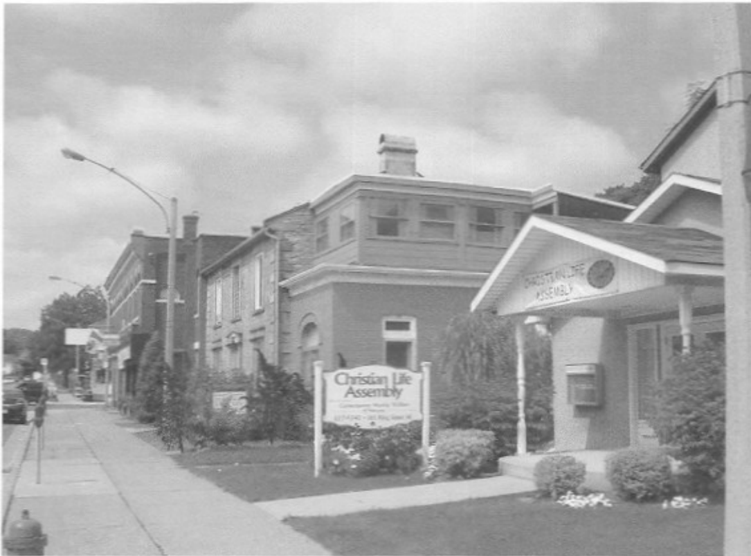
Figure 3: Traditional Architectural Detailing
